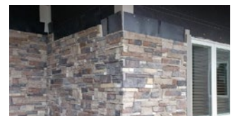
Corner Detail, Mid-installation
